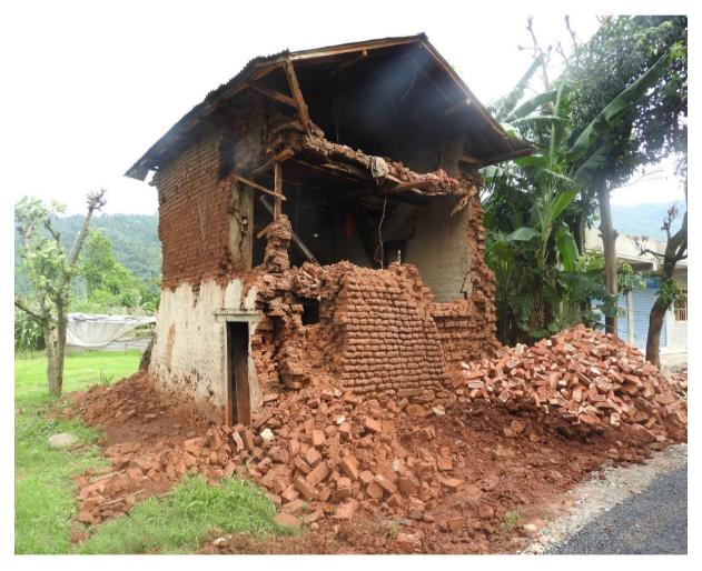
A brick-in-mud house in Bidur Municipality, Nuwakot that suffered damage during the earthquake.
